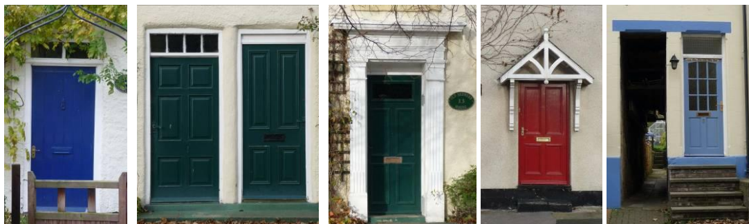
Plate 27. A selection of doors from the Green character area. (i) A tongue and groove board door typical of basic Victorian doorways and earlier Georgian styles. The overlight is Victorian in style. (ii) a pair of doorways, possibly once access to the residence on the left with the overlight and a passage to the rear on the right, but both now domestic. The six panel door is a modern reproduction of a Georgian style and the four panel door a Victorian style. (iii) a Tuscan door surrounding a modern door at no. 13 High Street (iv) a Victorian 4 panel door on Bank Top and another pair of twin doorways, this time Victorian but with a modern door replacement on Palmers Terrace.
