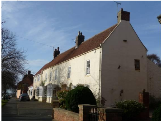
Plate 11. The Old Brewery House and neighbours with a typical 18 th century side elevation, modernised to the front c.1900
