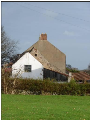
Plate 30. Town End Farm with stepped roof lines
