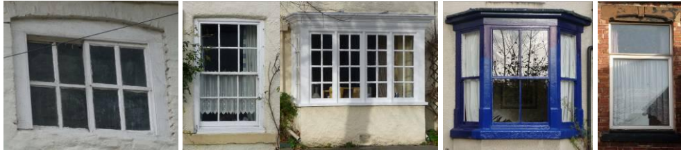
Plate 28. A selection of windows from The Green Character Area in broad chronological order. (i) a Yorkshire sliding sash window from the Manor House (ii) a 12 pane sash from 14 High Street (iii) a square bay from 13 High Street (iv) a Victorian bay from Bank Top and (v) a rear window opening with lintel detail on Kirtley Terrace (outside the Conservation Area) in a style used in the late 19 th and early 20 th centuries, but with a modern window.
