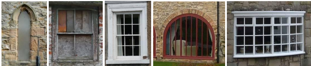
Plate 20. A selection of windows from the Church Street Character Area. (i) the church uses a mixture of 13 th century lancets and later 19 th century copies. (ii) derelict farm buildings retain some blocked up agricultural windows, but the entire range needs to find a new use. (iii) The Old Hall has 12 pane sash windows set within an architrave, typical of 18 th century styles. The conversion of former agricultural buildings has retained the hemmels to reflect the agricultural character, but other windows fit in less well with inaccurate modern pastiche.
