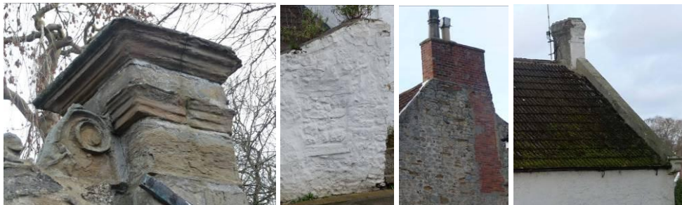
Plate 21. Small details indicating historic depth add to the interest of an area: (i) the ornate gate piers into the Old Hall, (ii) a blocked coal door in an outbuilding at the foot of Church Street, (iii) while historic character is often lost on the front of a house through the replacement of historic windows and doors with modern ones, great age can still sometimes be determined in the gable ends, (iv) many roofs are now covered in concrete tiles, but where water tabling and kneelers remain, historic character does too.
