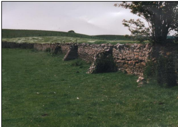
Plate 5. Remains of the deer park wall. This stretch is clearly in two phases, presumably the deer park wall has been lowered and rebuilt over the centuries (photo: John Smith, Bishop Middleham)
