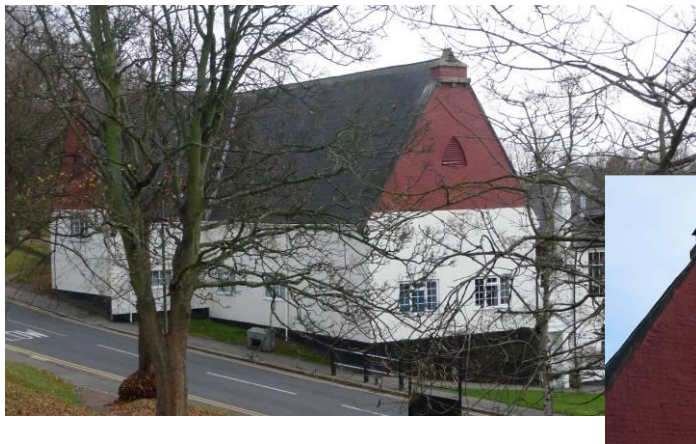
Plate 25. The Old School House and roofing detail; it originally had a bellcote
