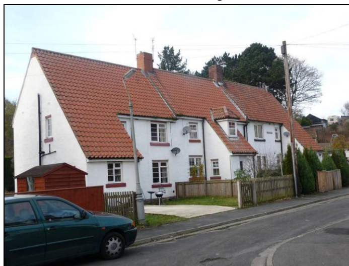
Plate 14. 1950s housing behind Church Street on Bishops Garth. Only no.3 retains its original horizontal metal glazing bars, probably purchased from Darlington which at that time supplied most metal windows in the UK.
