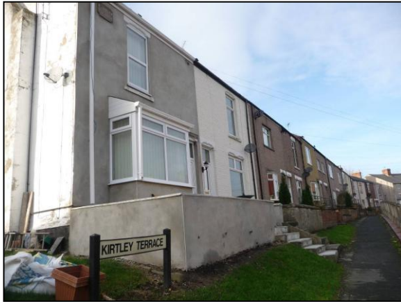
Plate 16. Early 20 th century terracing (this example outside the Conservation Area) has suffered from the loss of traditional features such as sliding sash windows and solid wooden doors with panelling. This is compounded by the use of wall coatings which do little to enhance the street and store damp problems for the future. On the plus side a number have retained detailing on the stone lintels and the old street name plate has survived on the end house below the eaves.
