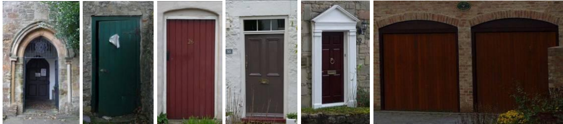
Plate 19. A selection of doors from the Church Street Character Area. (i) the 13 th century church doorway (ii) a simple ledged and braced door on an outbuilding (iii) a similar ledged and braced door now on a house (iv) a Victorian four panel door with overlight (v) a pastiche of a Georgian pedimented doorway with 6 panel door (vi) a modern double garage door – the use of brickwork and solid timber doors goes some way to making this development fit in.
